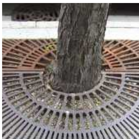
A 24" removable center ring is inserted to the grate to accommodate tree growth for a maturing tree.
