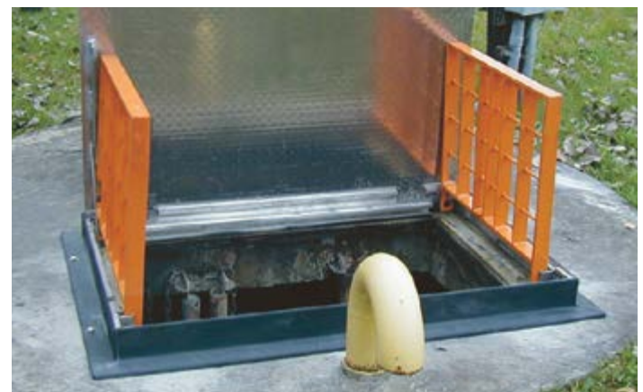
Open safety grates Safety orange painted aluminum grates provide a visual barrier around pit
