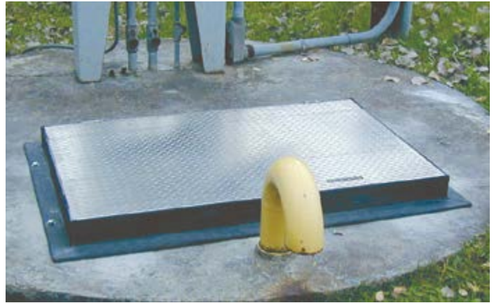
Aluminum 1/4" diamond plate cover with all stainless steel hardware
