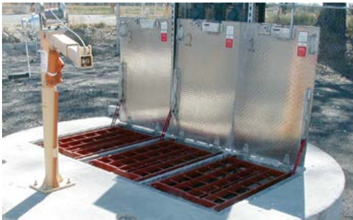
Open safety grates Safety orange painted aluminum grates provide a visual barrier around pit
