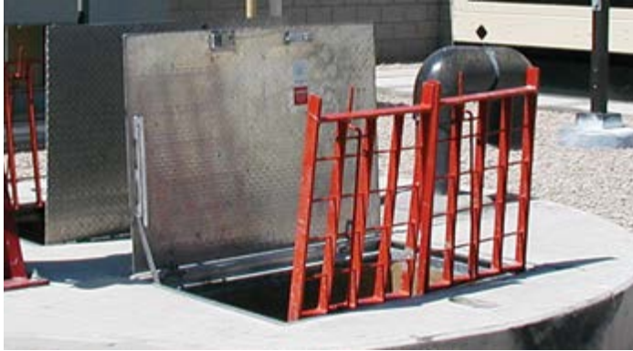
Closed safety grates Safety orange painted aluminum grates provide 300 psf non-traffic pedestrian rated fall through protection
