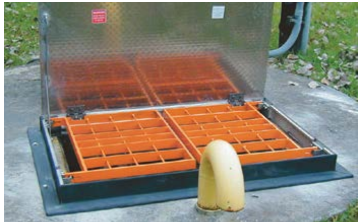
Closed safety grates Safety orange painted aluminum grates provide 300 psf non-traffic pedestrian rated fall through protection
